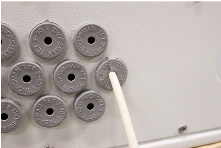
The photo shows the bottom of the control cabinet. Bottom side of control cabinet, communications cable installed:
