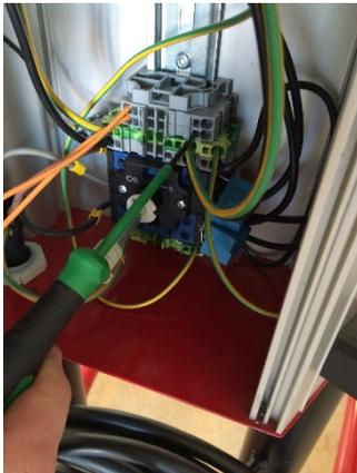
7. Install the cable from a potential-free contact to the terminals in the control unit.
